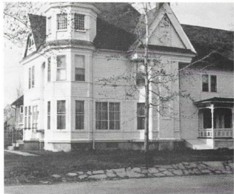
The convent was moved to its present site in Fall 1958 to make room for the new school. A foundation was dug that Winter while the Sisters stayed in another house on the property. (1978 photo from Sr. Monica)
